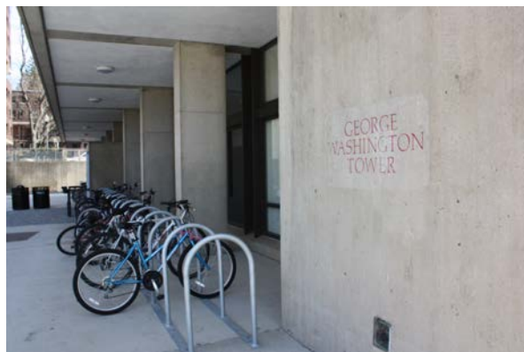
Photo: Pilotis 'lift-up' tower and shelter bikes 41
